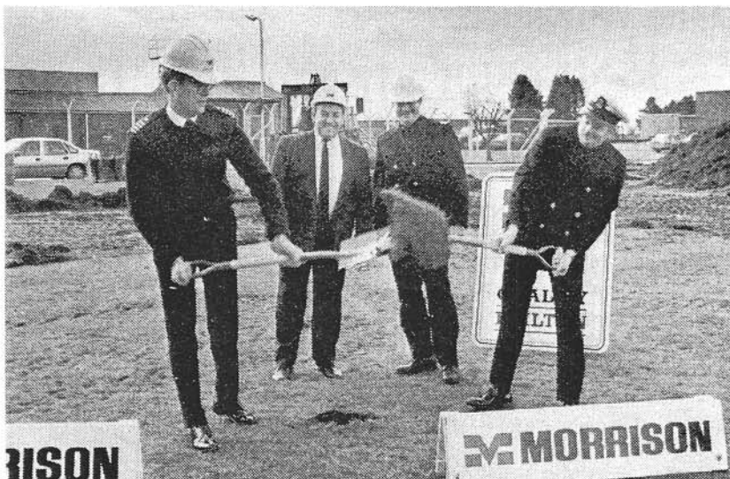
Capt. T.P. Lapierre and SHCM John Peterson, Navy Exchange Officer, officially broke ground on Feb. 5 for construction of NSGA Edzell's new Navy Lodge. The Lodge is scheduled for completion in 1993 and will contain 15 suites, each with its own kitchenette and bathroom facilities.
