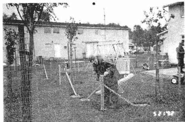
CE3 Don Miller doing the finishing touches on the fences.
