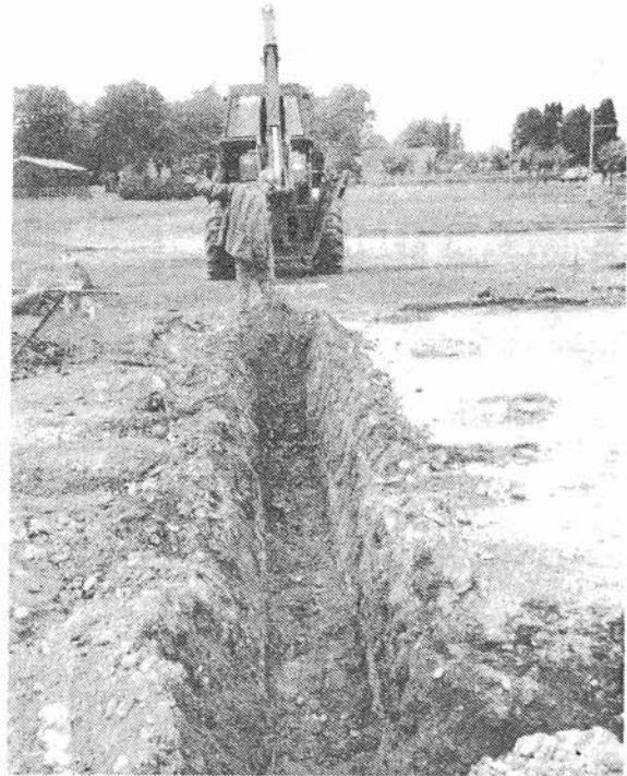
Equipment Operators digging the footers of the gas station project.
